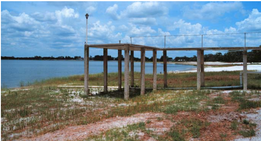
Figure 7-20. During periods when lake surface levels are low, natural system and cultural values associated with Lake Lotela are diminished.
