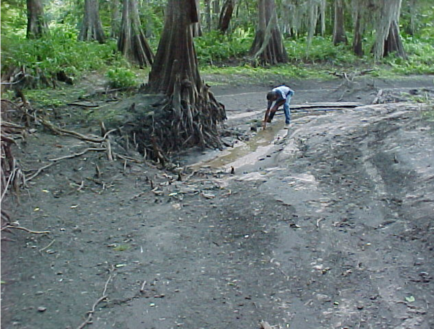
Figure 7-17. Peace River flowing into sinkhole near Bartow Wastewater Treatment Plant, May 2001.
