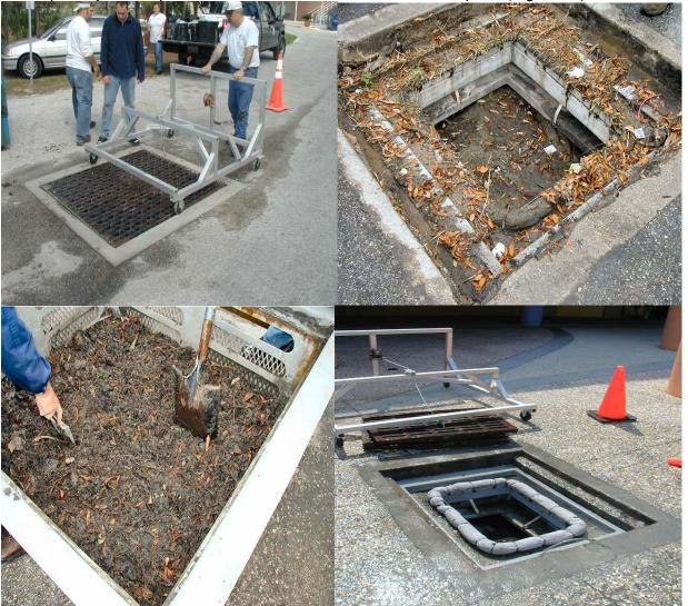
Figure 26. Cleaning out the skimmer box inserts. a) Crane being moved into place to remove the grate. b) Uncovering the mess that is inside. c) Pushing all the material into the basket and mixing it well in preparation to taking samples to send to the lab. d) Installing cleaned out basket and new boom to make ready to replace the grate (photo credits: Suntree Technologies, Inc).
