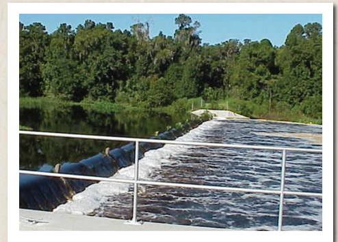
Wysong Structure with Main Gate Fully Inflated (Raised)
