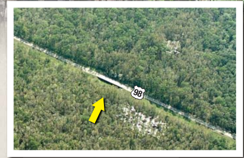
Aerial View of the US 98 Bridge Crossing on the Hillsborough River
