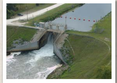
Inglis Bypass Structure
