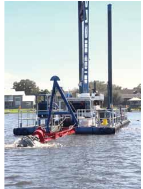
Dredging on Lake Seminole.
