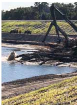
Water and muck slurry entering the dredge material management area.
