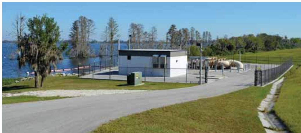
Lake Hancock Outfall Treatment Facility.
