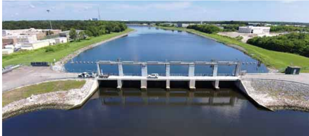
Tampa Bypass Canal Structure S-160.
